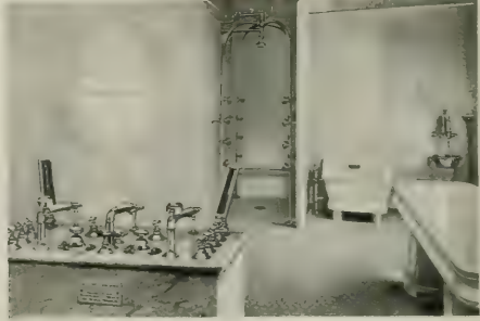
Hydratic Douche Room, Charles B. Towns Hospital.
